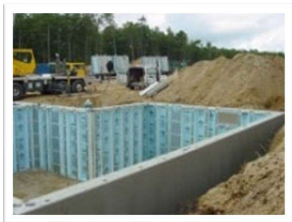
Fig. 14.17 Precast Concrete Foundations
