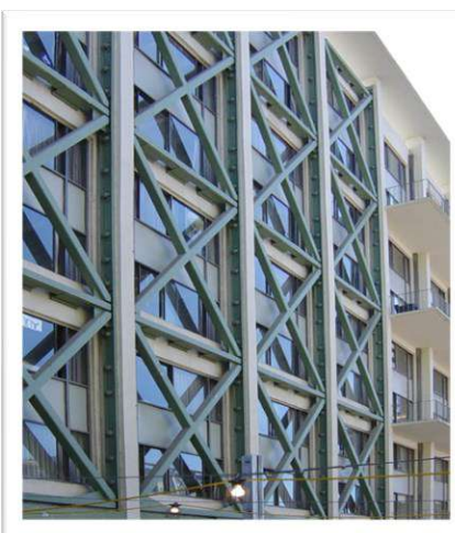
Fig. 14.12 Supplementary damper
