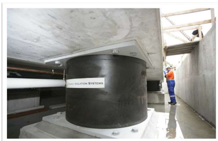
Fig. 14.11 Base isolater
