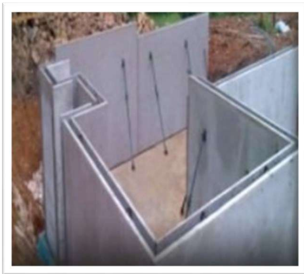
Fig. 14.18 Twin Wall Technology
