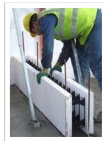
Fig. 14.19 Insulating Concrete Formwork
